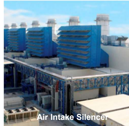
Gas Turbine & Acoustic Package
